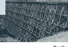
**Trestle**: an open framework used to support an elevated structure such as a bridge
